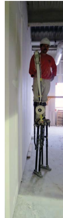
Taping the drywall.
