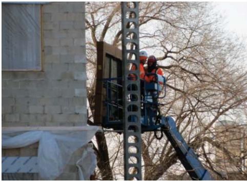
Windows being delivered to second floor.
