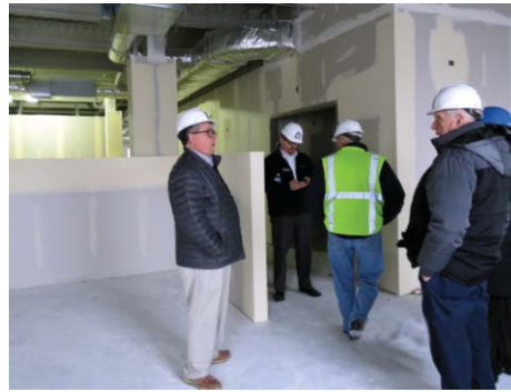
Second floor ready for paint.
